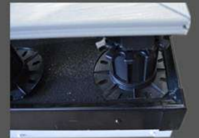
Pedestals running along an edge of an elevated area (flat roof, balcony or terrace) have edges that can be broken off to create straight edges
