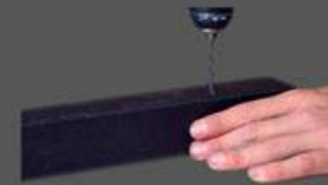
Pilot hole composite bearers before fixing pedestals
